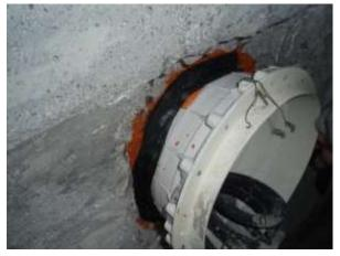
3. Repairing and waterproofing of honeycombed areas, tie holes and pointing applications, with the crystalline waterproofing system of the liquid applied PENETRON<sup>®</sup> and the repairing PENECRETE MORTAR<sup>®</sup> and repair of cracks with running water with the crystalline waterproofing rapid set waterplug PENEPLUG<sup>®</sup>.
