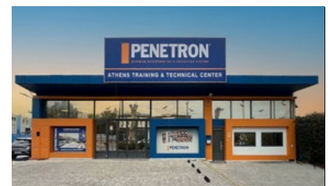
PENETRON HELLAS Facility, Athens, Greece
