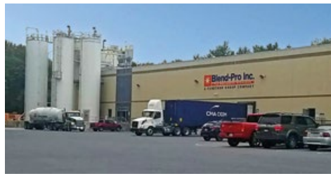
Penetron/Blend-Pro Manufacturing Facility, Allentown, Pennsylvania, USA
