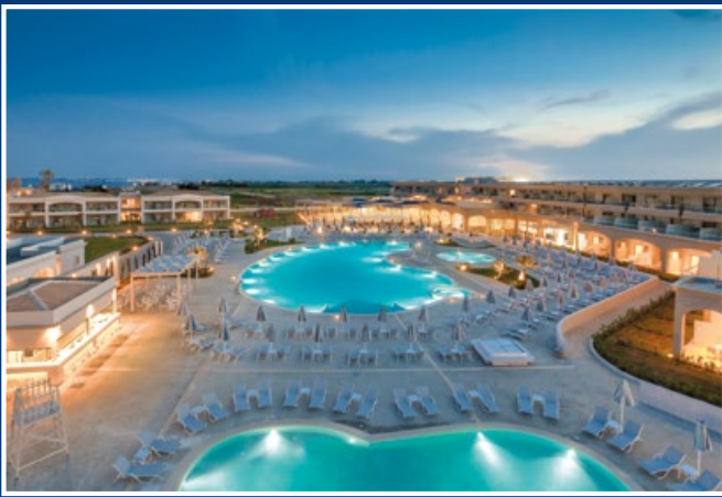
SWIMMING POOL SYSTEMS
