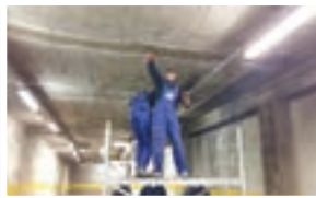
Application of PENETRON® INJECT, integral crystalline crack-injection system
